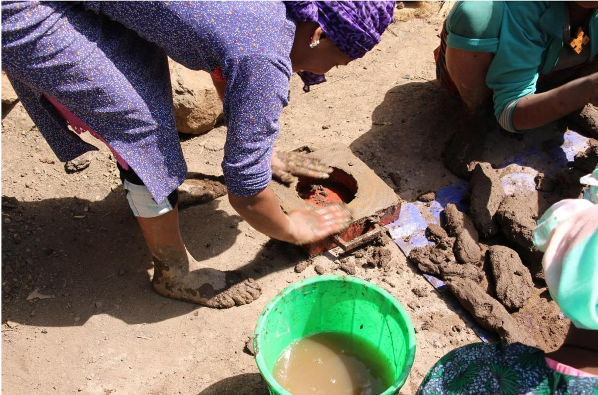
Making clay-bricks for the chimney with special molds
