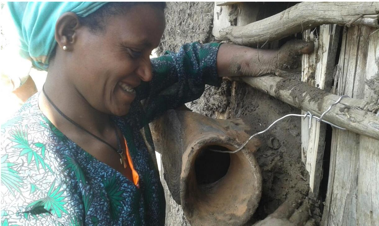
Fixing the outlet outside of the house wall
