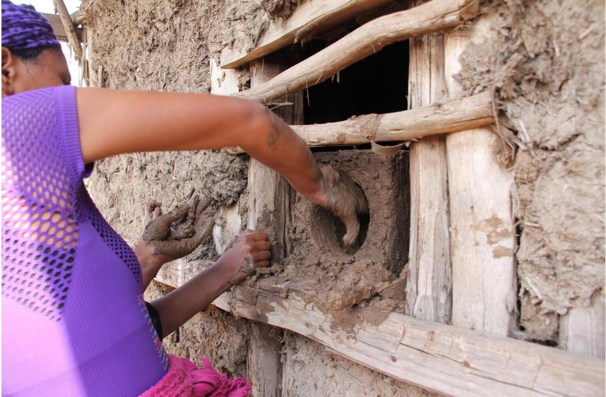
Making the hole through the housewall to fix the outlet
