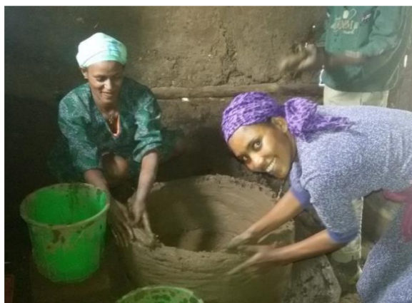
Genet und Yeshwa building a stove
